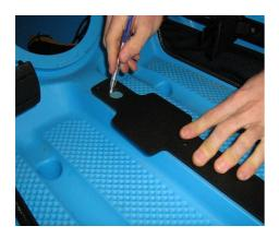
§ Using the 20mm gland hole on the plastic base as a guide scribe cable outlet position.
